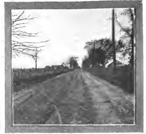
Showing a fine stretch of road near Lacolle after scraping
